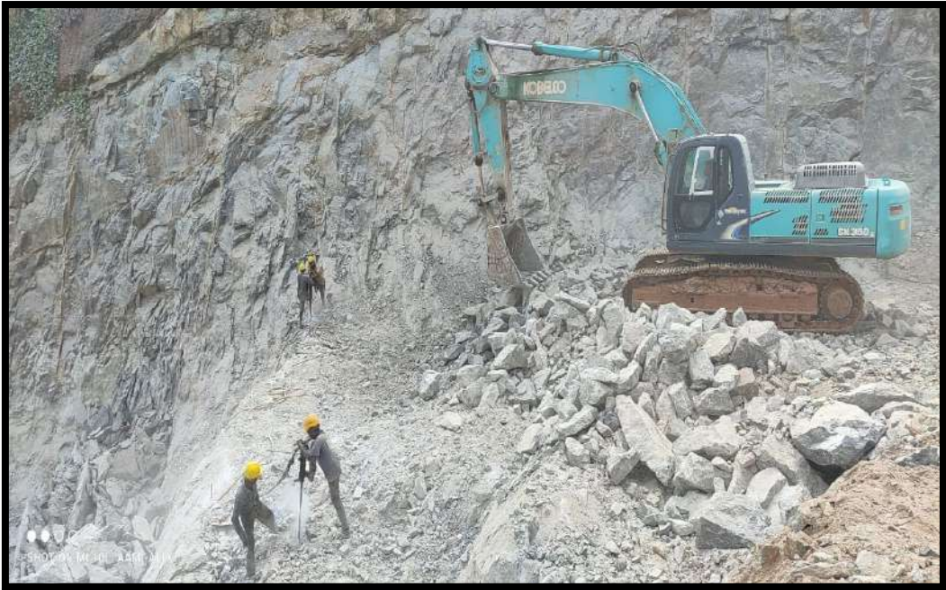
Workers with personal protective equipments
